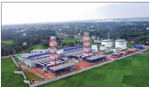
Power Pac Mutiara Jamalpur Power Plant.
