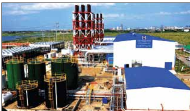
Dutch Bangla Power Associates Ltd.
