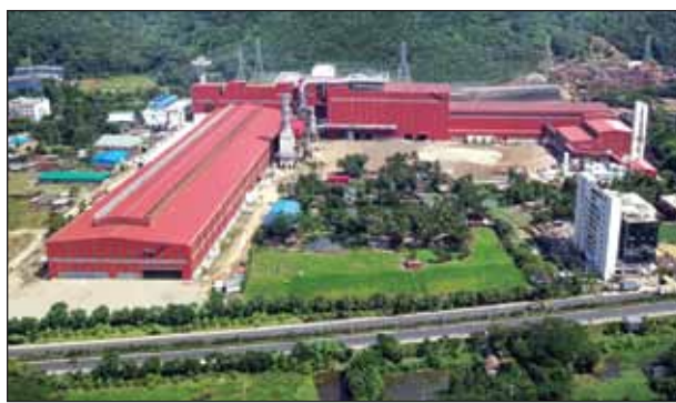
GPH Ispat (New Project)
