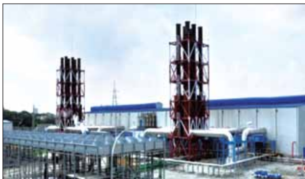
Orion Power Meghnaghat Ltd.
