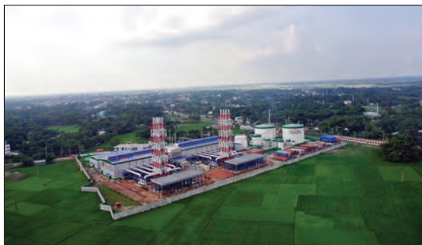
Power Pac Mutiara Jamalpur Power Plant.
