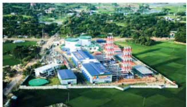
Power Pac Mutiara Jamalpur Power Plant Ltd.
