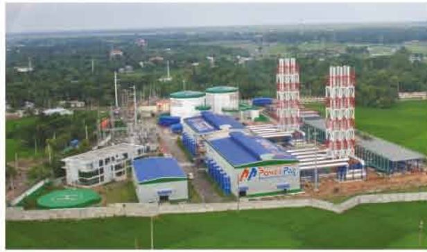
Power Pac Mutiara Jamalpur Power Plant Ltd.
