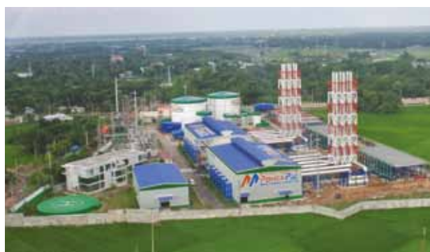
Power Pac Mutiara Jamalpur Power Plant Ltd.
